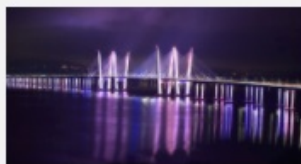
Governor Mario M. Cuomo Bridge in New York
